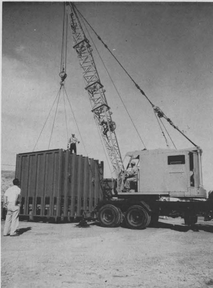
**FIRING CHAMBER** for explosives is unloaded at Livermore's Site 300. The 20-ton chamber was fabricated of armor plate by Todd Shipyards, Alameda, Calif. at a cost of \$16,600. Watching the unloading (left) is Howard Cole, Test Operations Section (8121-2), whose organization will use the firing chamber at the site.
